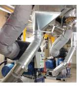
Robox Screw for the fluidisation air for its yeast fermenter
